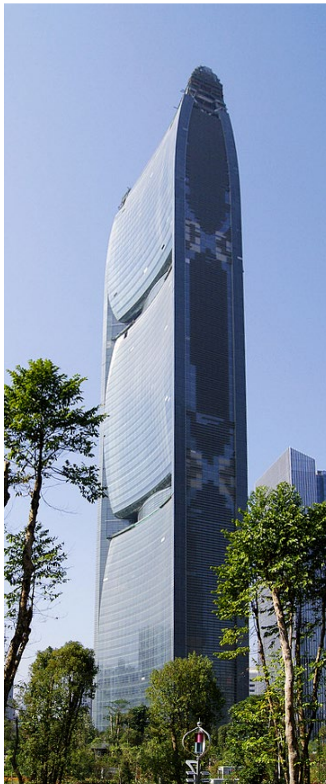
Pearl River Tower - New office of the China National Tobacco Corporation. By Brad Wilkins. Source: CC BY-SA 3.0"
