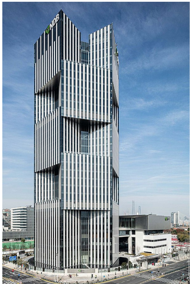
New Development Bank (BRICS Bank) headquarters in Shanghai, China Source: By Donnie28. CC BY-SA 4.0
