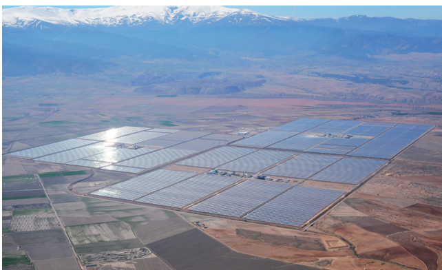
Thermal energy storage. Source: Kallerna/ Wikipedia Commons/ CC 4.0
