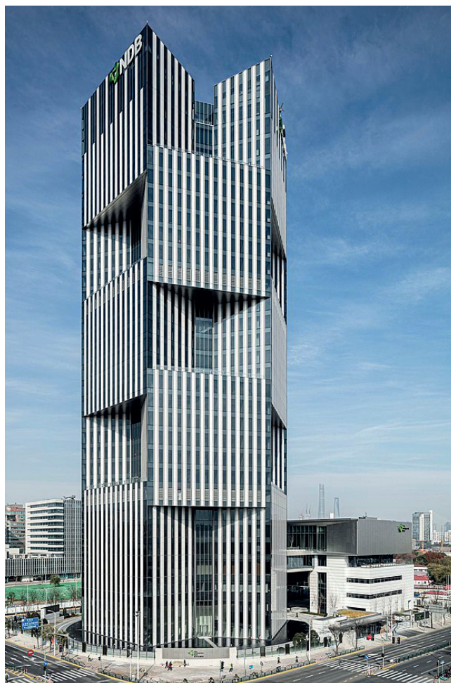
New Development Bank (BRICS Bank) headquarters in Shanghai, China Source: By Donnie28. CC BY-SA 4.0
