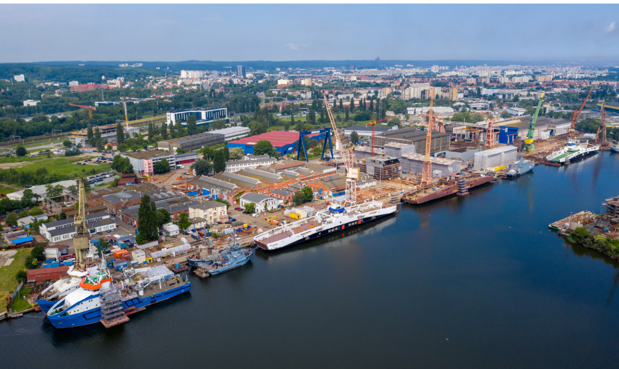
Remontowa Shipbuilding Shipyard with Ro-ro vessels under construction
