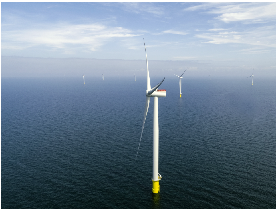
Photo 6 – Kriegers Flak Offshore Wind Farm, Source: Vattenfall AB
